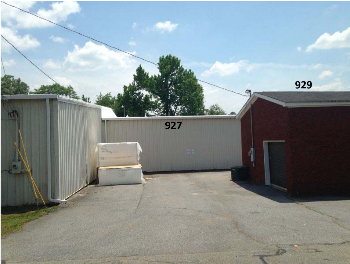
VIEW FROM MIMOSA LANE TO REAR OF 929 BUILDING AND SIDE OF 927 BUILDING
