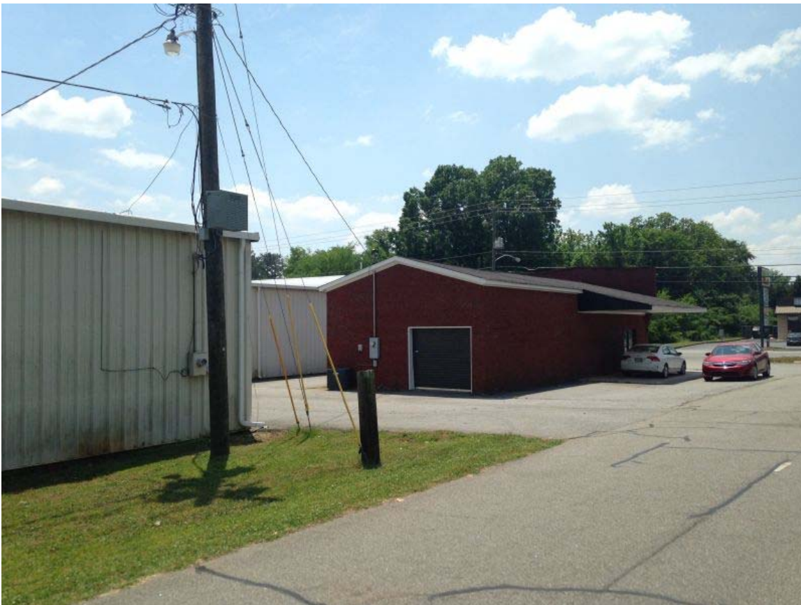
VIEW FROM MIMOSA LANE TO REAR OF 929 BUILDING.
